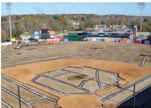
▲ Top: THE STRATEGY PLAN for the Lakes Community HS football field. Bottom: INSTALLED DRAINAGE at Fifth Third Stadium, home of the West Michigan Whitecaps.
