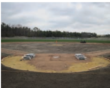
>> Above left: CLAY BRICKS were installed in the pitcher's mound and home plate.
