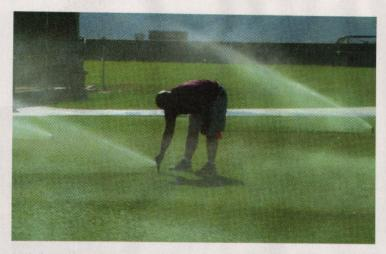
mainline hoop supplies the water from the pump house. Each field then has a 3-inch mainline loop that provides water to two 12-inch valves. Each field has a 3-inch master valve and the ability to isolate any of the 12 valves and still supply water to the rest of the field. Each playing field is equipped with an average of 90 sprinkler heads and 10 1 1/2-inch quick couplers. The Campus is a Hunter irrigation facility, Kennedy says.
