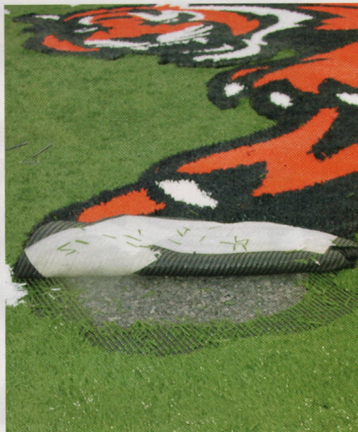
Installation of a special logo on a synthetic field. Photo by Darian Daily.
