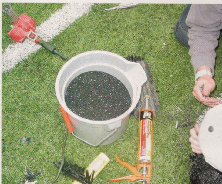
Rubber mix used for resiliency on synthetic fields. Photo by Darian Daily.
