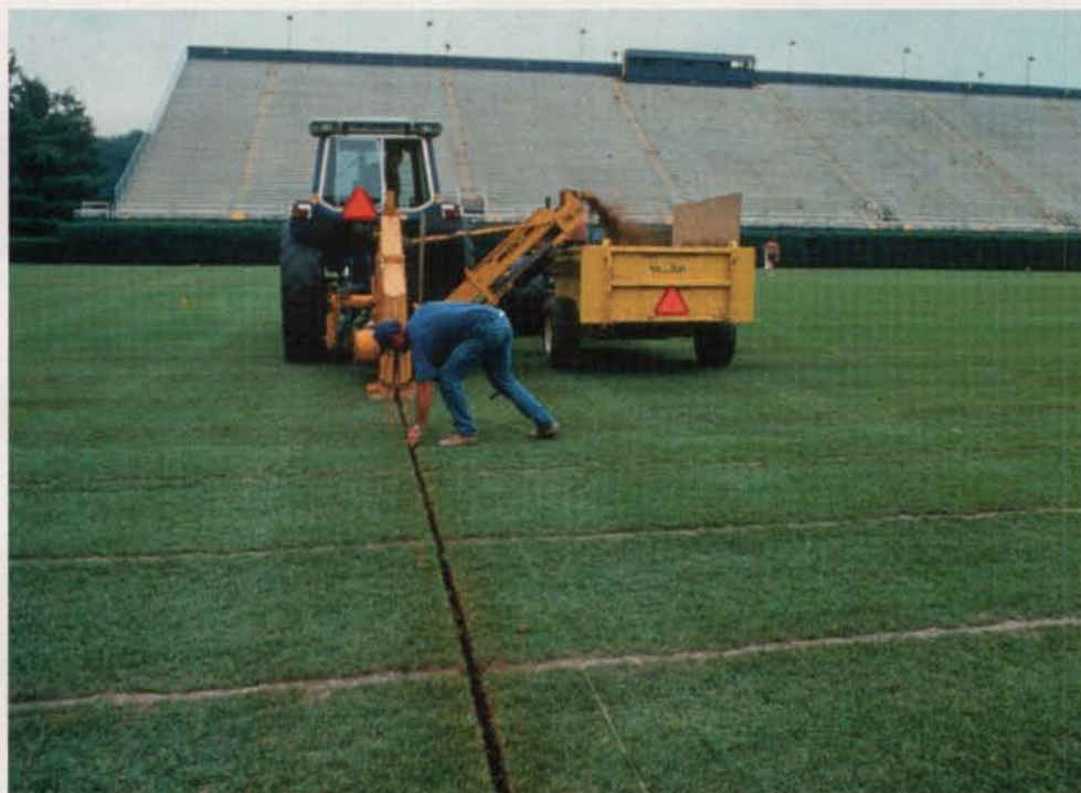
Installing a grid drainage system.
