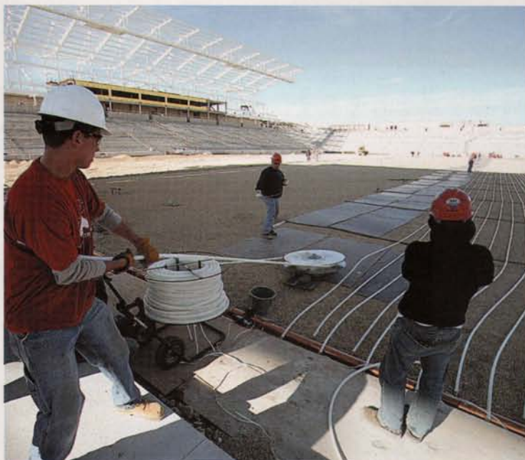
Motorized sled, custom-made for the project by Althoff Industries, carried the loops of PEX tubing from one end of the playing field to the other.
