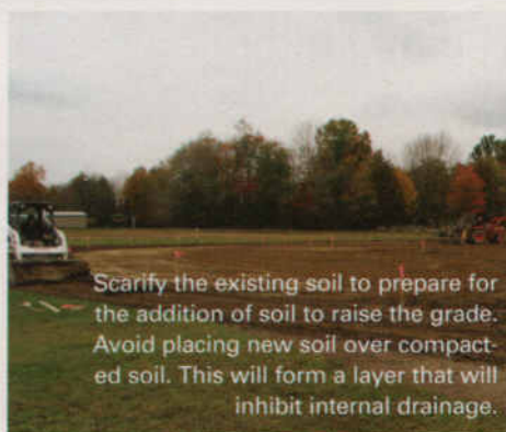
Topsoil and skinned area soil is brought in so the final grade can be set. Grade and scarify the soil in preparation for seed, sprigs, or sod.
