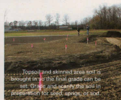
Scarify the existing soil to prepare for the addition of soil to raise the grade. Avoid placing new soil over compacted soil. This will form a layer that will inhibit internal drainage.
