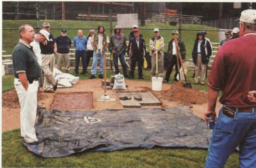
Dave Runkle of Luck Stone and Mark Roberts of Herod Seed demonstrated rebuilding batter's boxes and pitchers mounds with bag clay vs. clay bricks.
