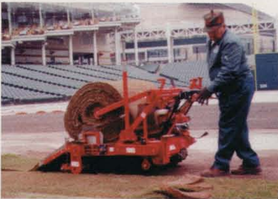
INSTALLED CLEVELAND INDIANS IN 42" AND 48" ROLLS
