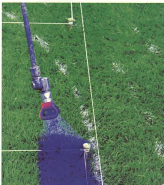
Paint should be applied at a recommended spread rate by spray, brush or roller.
