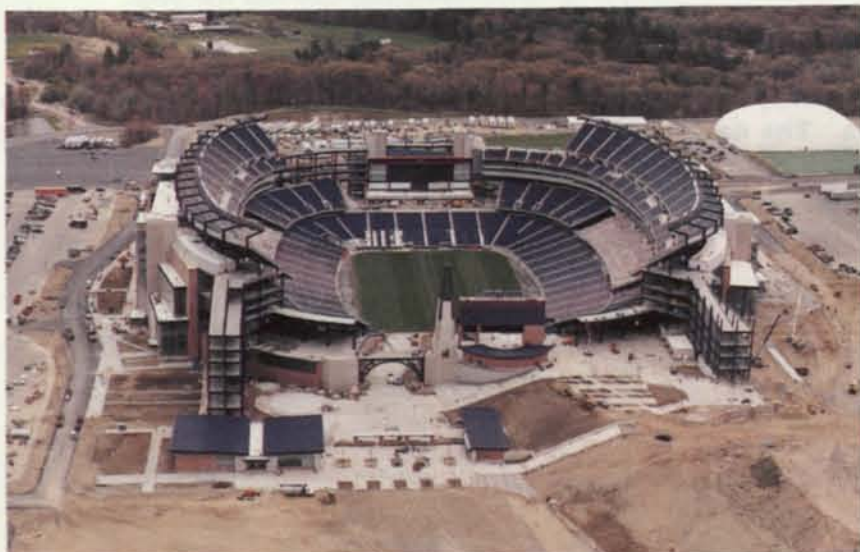
The Patriots' new radiant heating/turf warming system uses 29 miles of cross-linked polyethylene (PEX) pipes that warm the soil.
