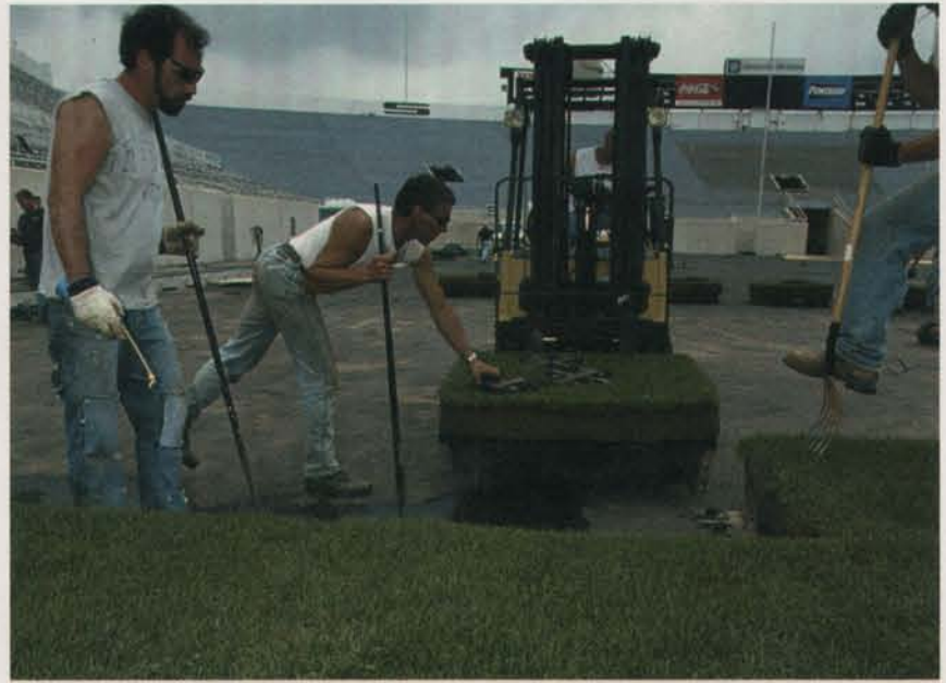
The modules were placed in the same order that they occupied at the Hancock Turf Center so that the edges and seams fit back together tightly.
