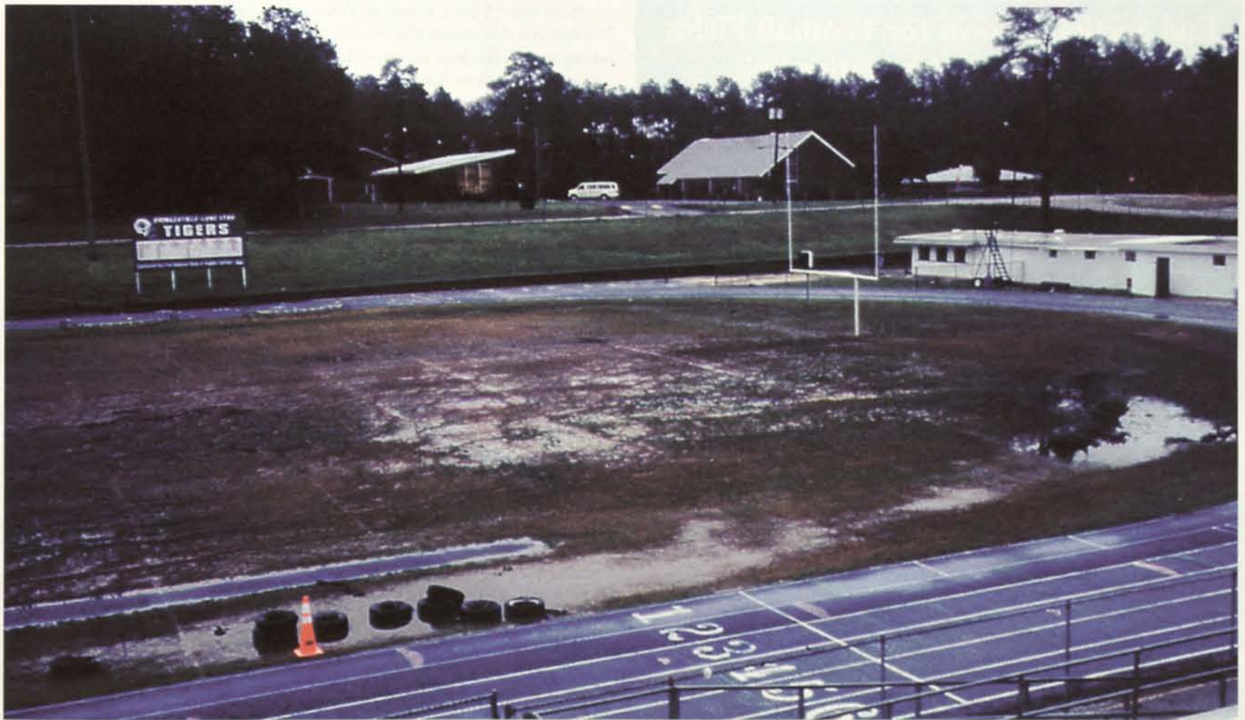
Unfortunately, too many athletic fields are constructed without an installed internal drainage system and don't have adequate crowns to rapidly remove excess water.
