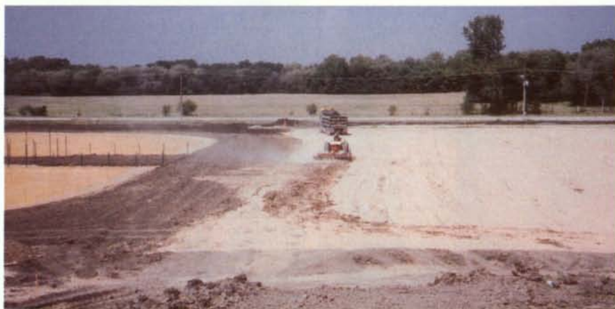
In the combination softball outfield and soccer field, calcined clay was incorporated into the soil to a depth of four to six inches.
