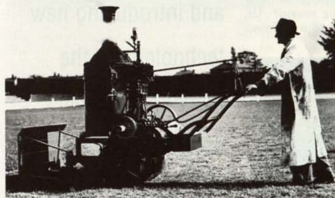
A Leyland steam-powered mower designed for sports turf.
