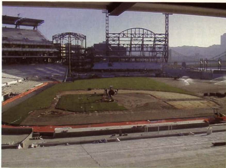
A view of the field, only halfway covered with sod
