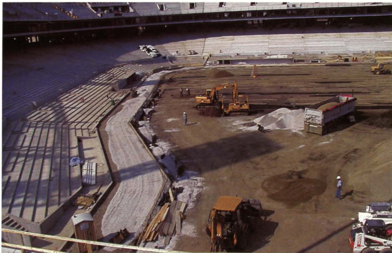
A solid foundation is important to quality turf. Here, workers prepare the soil mixture on which the sod will be laid.
