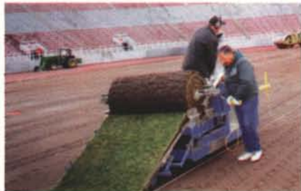
INSTALLED OHIO STATE (AND STRIPPED) 2" THICK TURF 48" ROLLS
