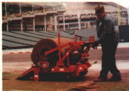
INSTALLED CLEVELAND INDIANS IN 42" AND 48" ROLLS
