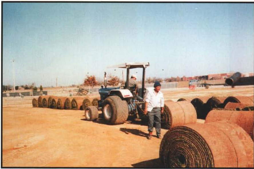
A machine maneuvers heavy big-roll sod pieces into position. Courtesy: Don Uber
