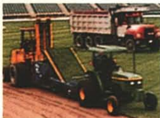
Stripped and installed Jacobs Field Cleveland Indians
