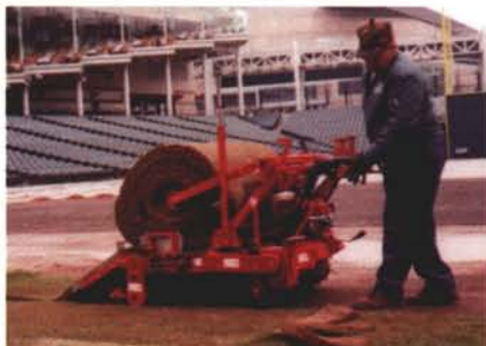
INSTALLED CLEVELAND INDIANS IN 42" AND 48" ROLLS
