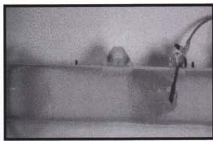
The Toro NutriFlow Fertigation system uses an injector quill to distribute nutrients evenly into the lines of an installed irrigation system.
