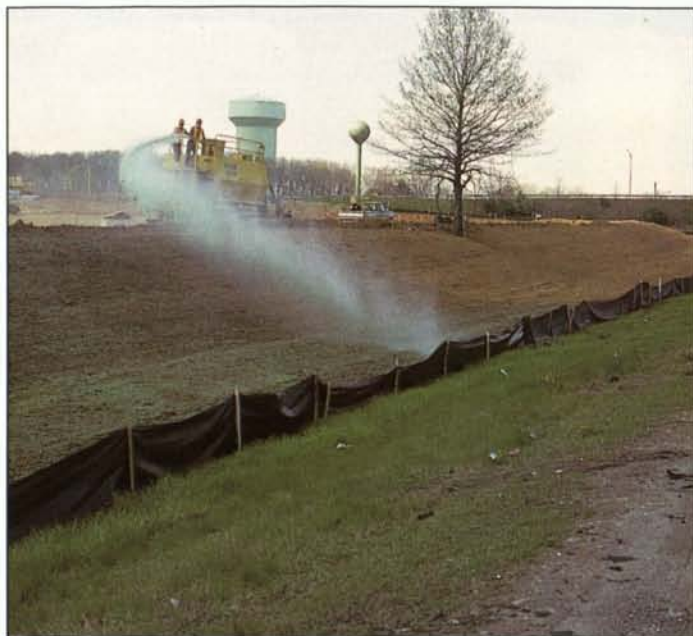
Hydro-applications are a practical solution for large areas of bare ground and for remote or limited access sites.
