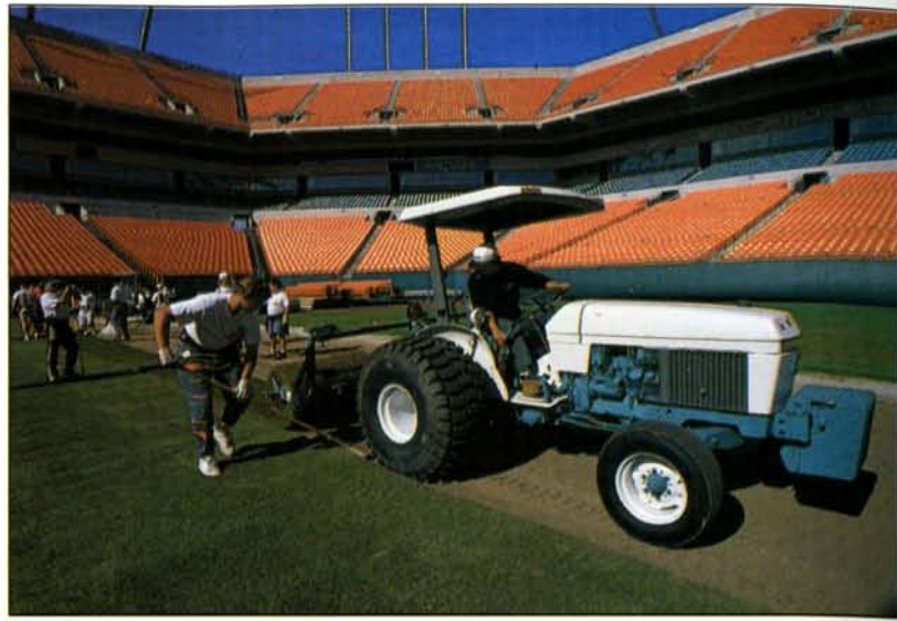
Big-roll sod is preferred over slabs and small rolls because there are fewer pieces involved and fewer edges. Photo courtesy: West Coast Turf.
