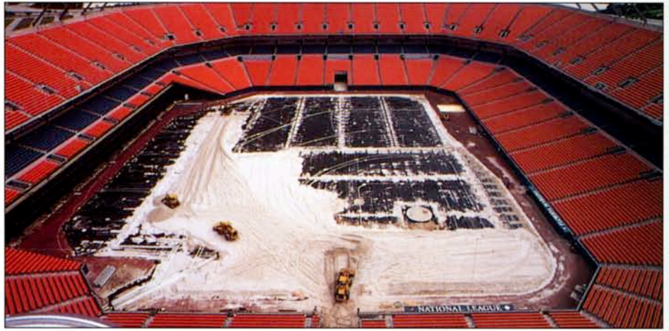
Joe Robbie Stadium undergoes sand profile distribution, covering drain lines and irrigation lines. Photos courtesy: The Motz Group and Deborah Gray Mitchell.
