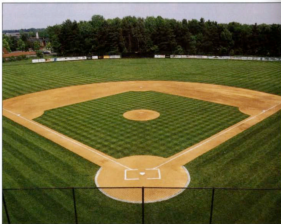
The baseball diamond at Boardman High School, now known as Dave Dravecky Field, has been reconstructed to eliminate structural defects like the depressed infield of the original facility. Photo courtesy: Jim Puhalla.
