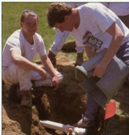
Undergraduate technology students Tom Welch (left) and Rus Myers install a valve manifold on SUNY-Cobleskill's soccer field as part of their class project to design and install an automated irrigation system. Photos by George Crosby.
