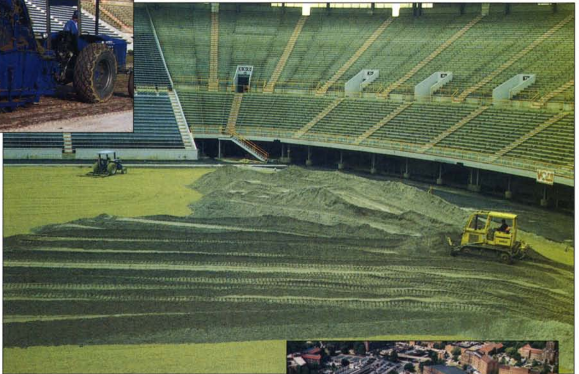
Nutri-Turf sprigged Neyland Field with Tifway 419 (top). The rootzone consists of 90% sand and 10% reed sedge peat. Neyland Stadium in days of artificial turf (right).
