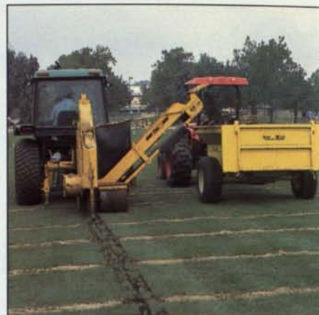
Installation of the sand-conduit drainage system, July 1994.
