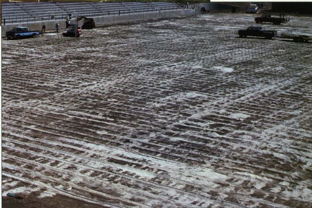
Construction of the soccer/football field at Cal State University Fullerton in 1991. After laying a half-inch of sand, the entire field is sodded. (Photos courtesy of Cal State Fullerton.)
