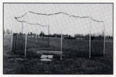
can be set up in less than ten minutes. The cage's poles are set into one-footdeep sleeves that have been set in concrete. The sleeves have locking hasps so that the poles can only be removed by authorized personnel.
