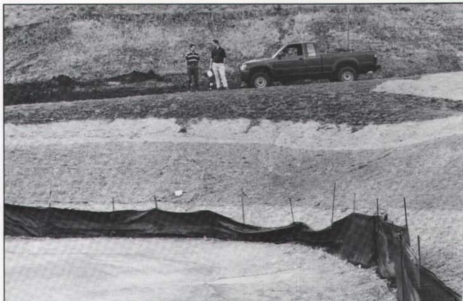
Superintendent Sean Hoolahan (r) and Gilbert Araki from Pacific Agricultural Sales look over green protected by blankets and silt fence.
