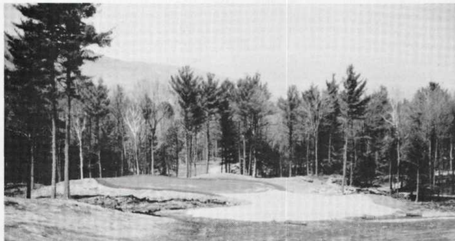
The fairways were capped with six inches of sand to improve drainage and speed establishment of the bentgrass.
