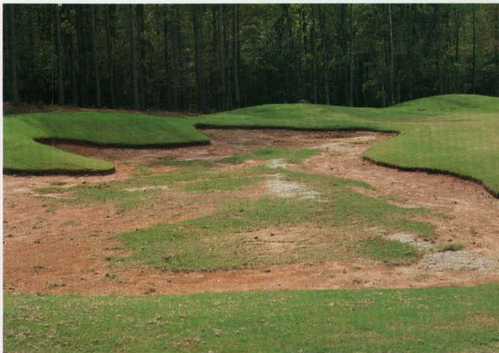
Bunker sodded and ready for sand.
