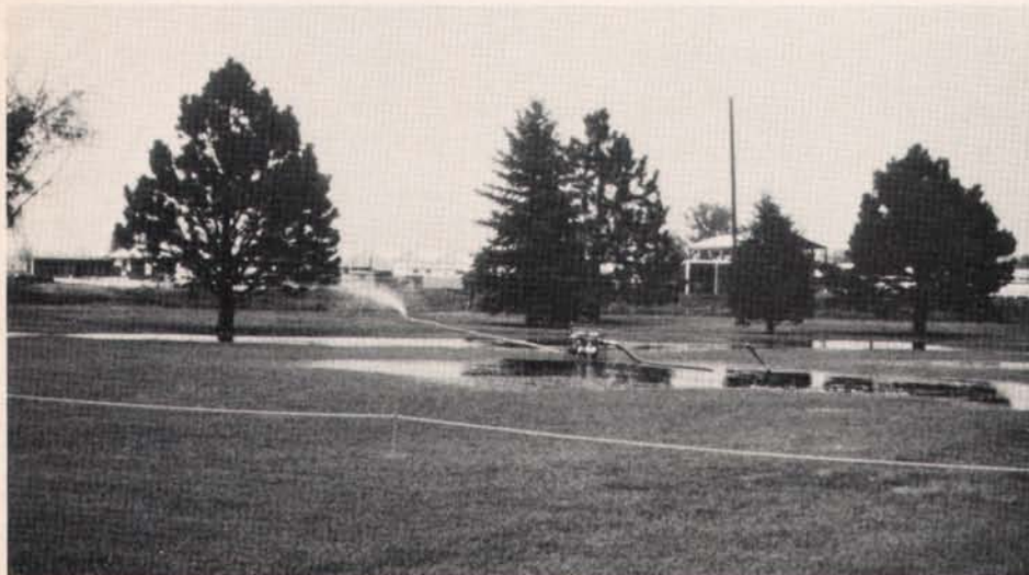
Sump pumps were used frequently to remove surface water from low spots before drainage was installed.
