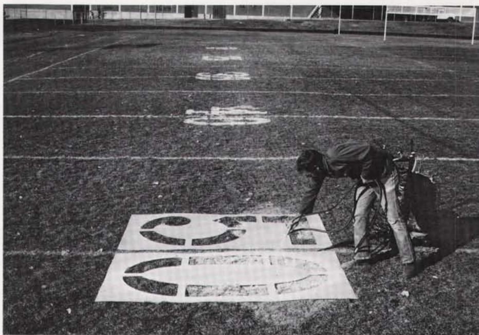
Using stencil to paint numbers on football field. Photo courtesy: Newstripe, Inc.
