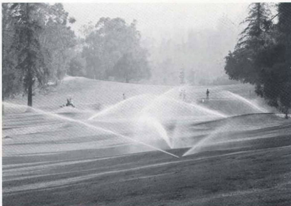
Syringe cycles can be activated by a button on the field station, from the central controller, or with a hand-held remote radio.
