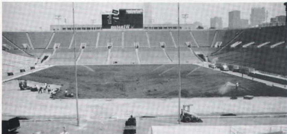
Temperatures soared during the three days the sod was installed.
