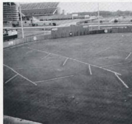
Drain network in left field backfilled with sand.
