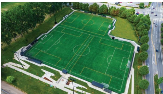
Topaz Park: Finlayson Field , Victoria, BC, Canada — GPM Civil Contracting Incorporated
