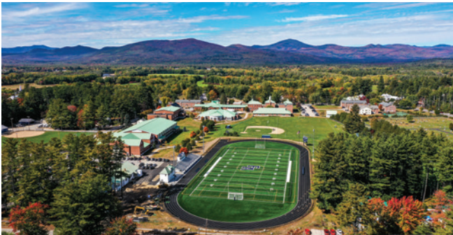
Atwood Stadium at Fryeburg Academy , Fryeburg, Maine — Activitas Inc.
