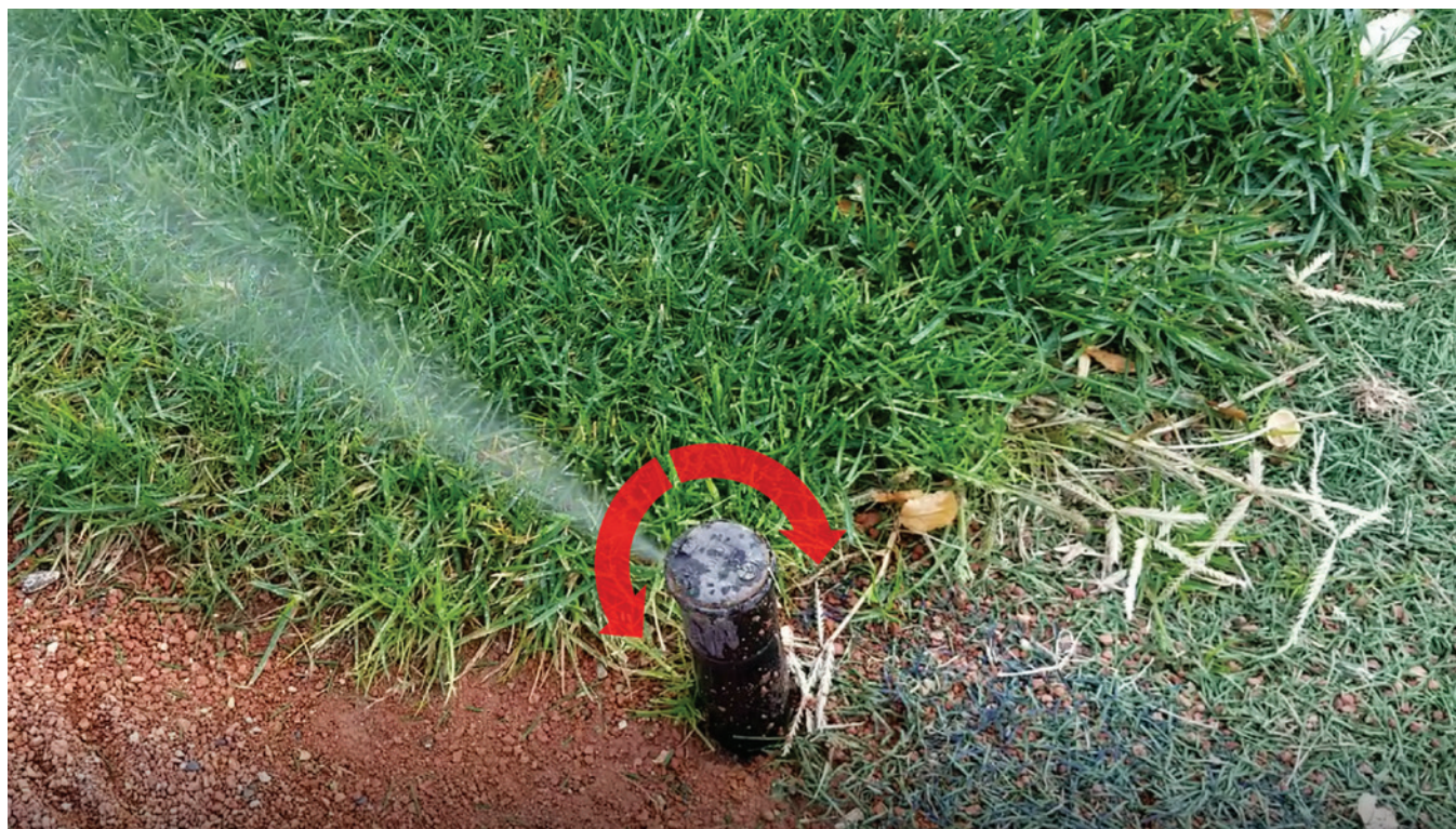
Figure 2: Sprinkler head spinning too fast from too high pressure air and/or too little water in lines.
