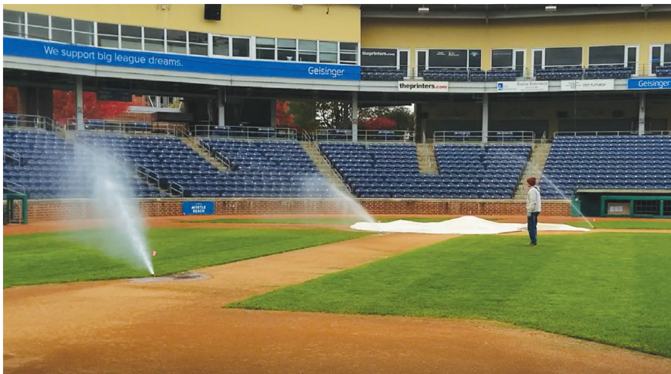
Figure 4. Example of sprinklers at different stages of the blow-out process.
