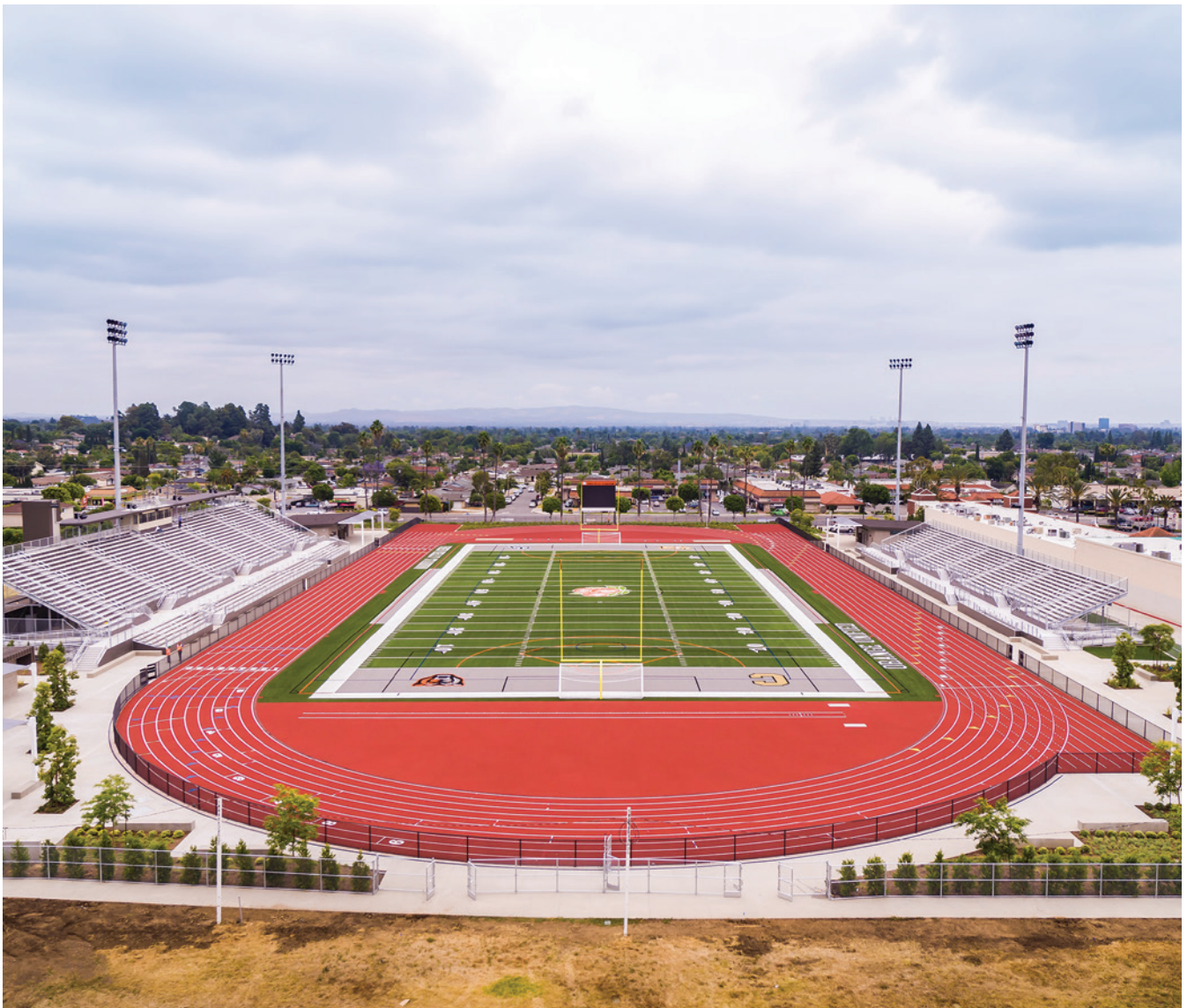
Photo courtesy of Byrom-Davey, Inc.
