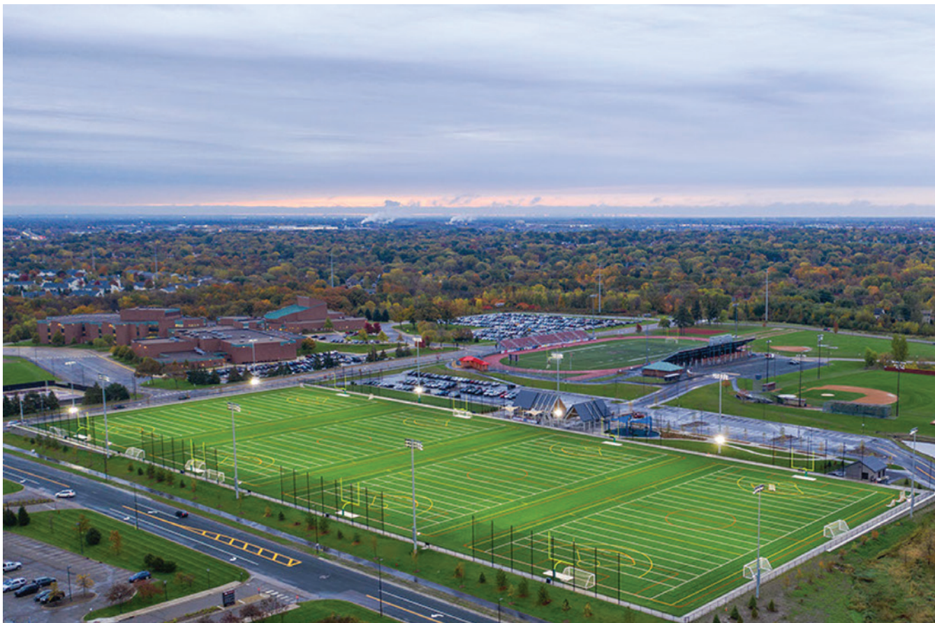
Photo courtesy of Stantec Sports Group
