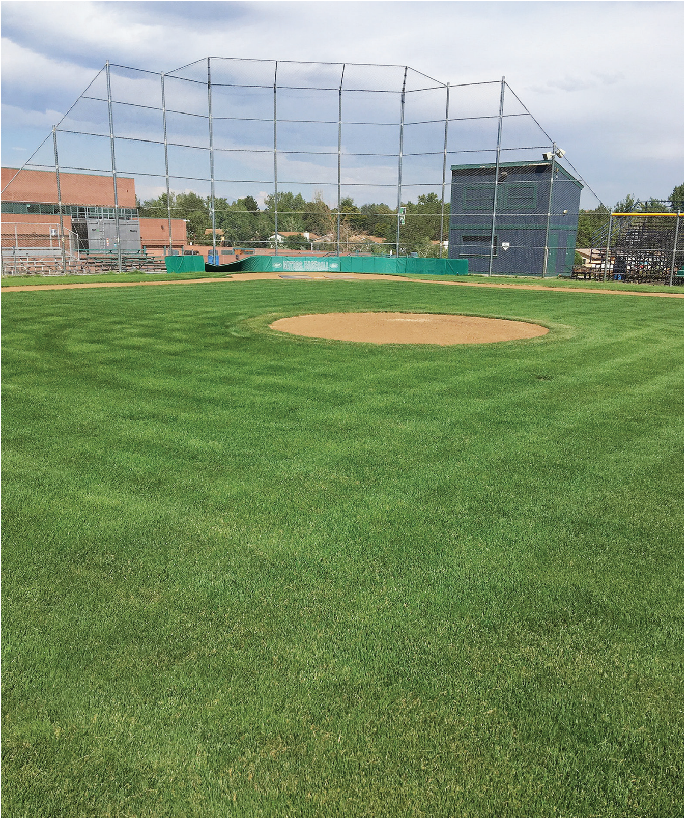
New sod installed along base paths, home plate circle and pitching mound. Existing infield turf was aerated and overseeded to improved density and uniformity.
