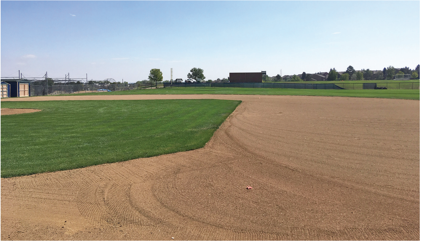
Infield graded and toppedressed to correct drainage
