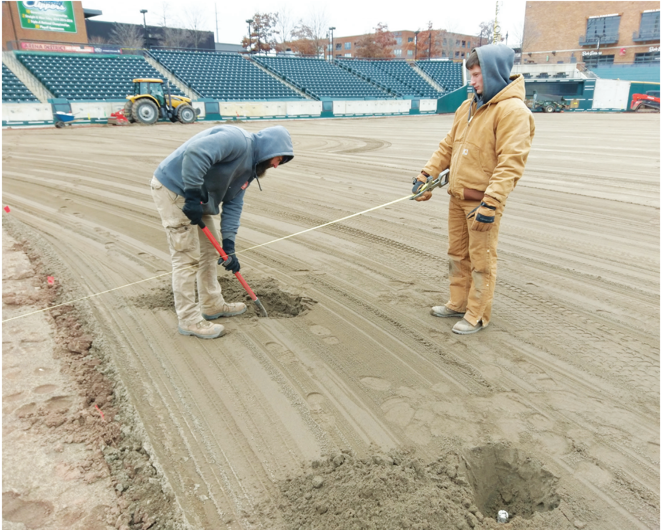
Irrigation heads were relocated to 4'6" off edges.
