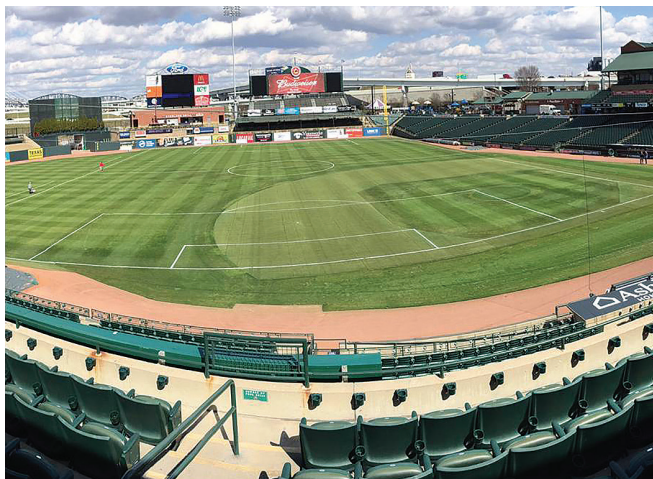
(Left) The day before the first soccer game. (Right) For soccer games the mound lowers into the ground and is leveled with foam and approximately 6 yards of sand. AstroTurf is then laid on top and pinned down.
