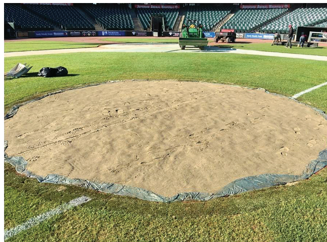
(Left) The day before the first soccer game. (Right) For soccer games the mound lowers into the ground and is leveled with foam and approximately 6 yards of sand. AstroTurf is then laid on top and pinned down.
