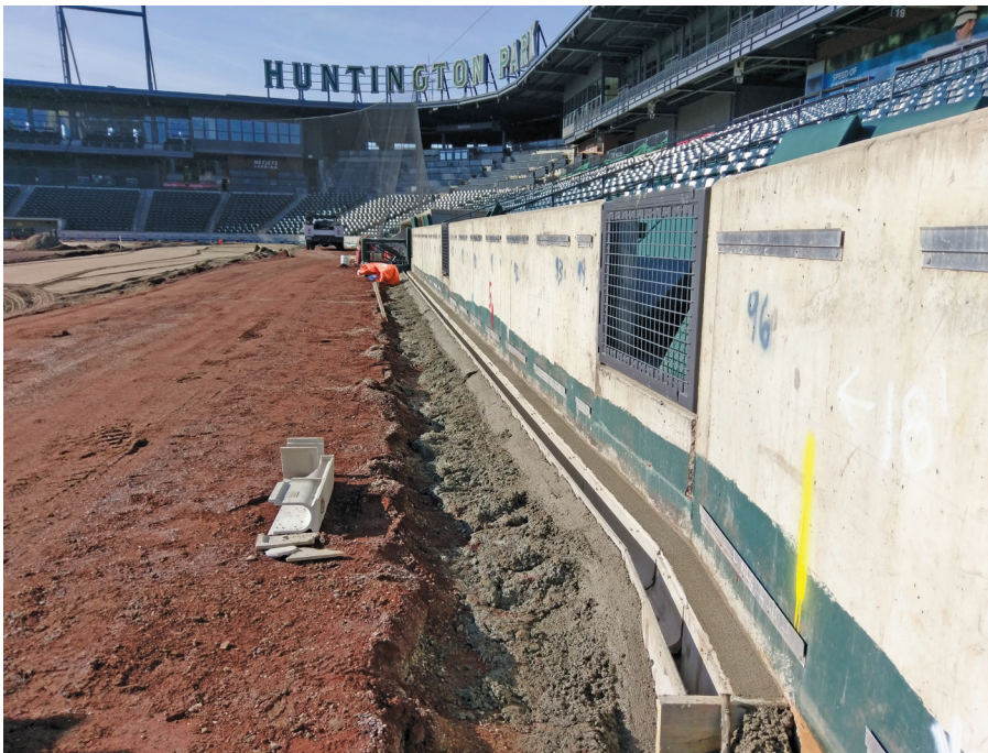
Trench drains getting finish concrete.
