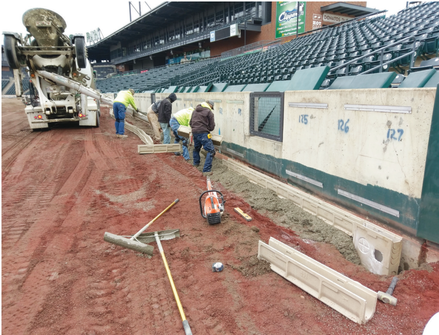
Trench drains being set by the concrete contractor.
