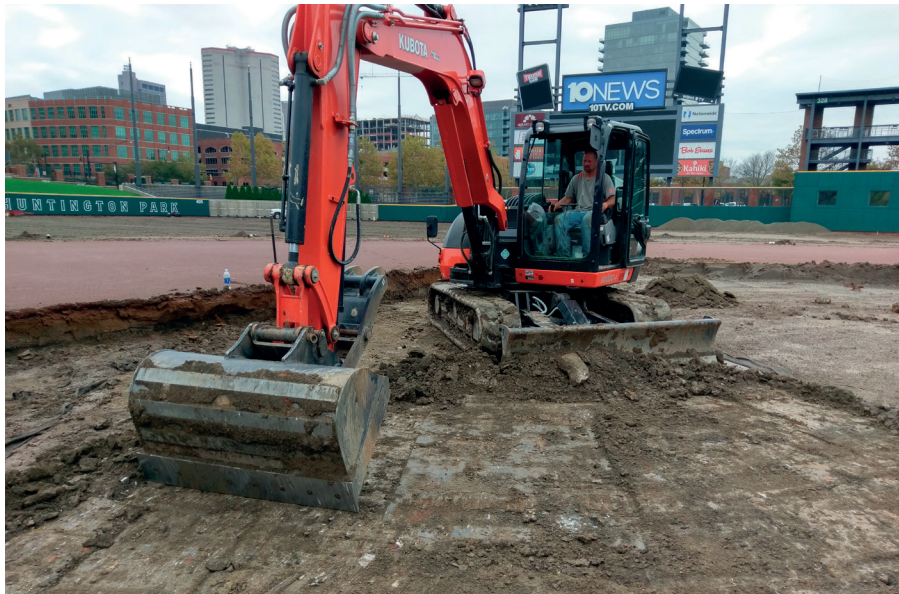
Jason Griffiths from Ag Design excavating subgrade material from the infield to drop the elevation.
