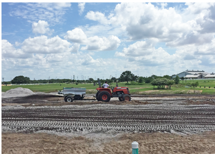
Amending the sand root zone of a new putting course with coffee grounds. Texas A&M AgriLife photo by Ben Wherley.
