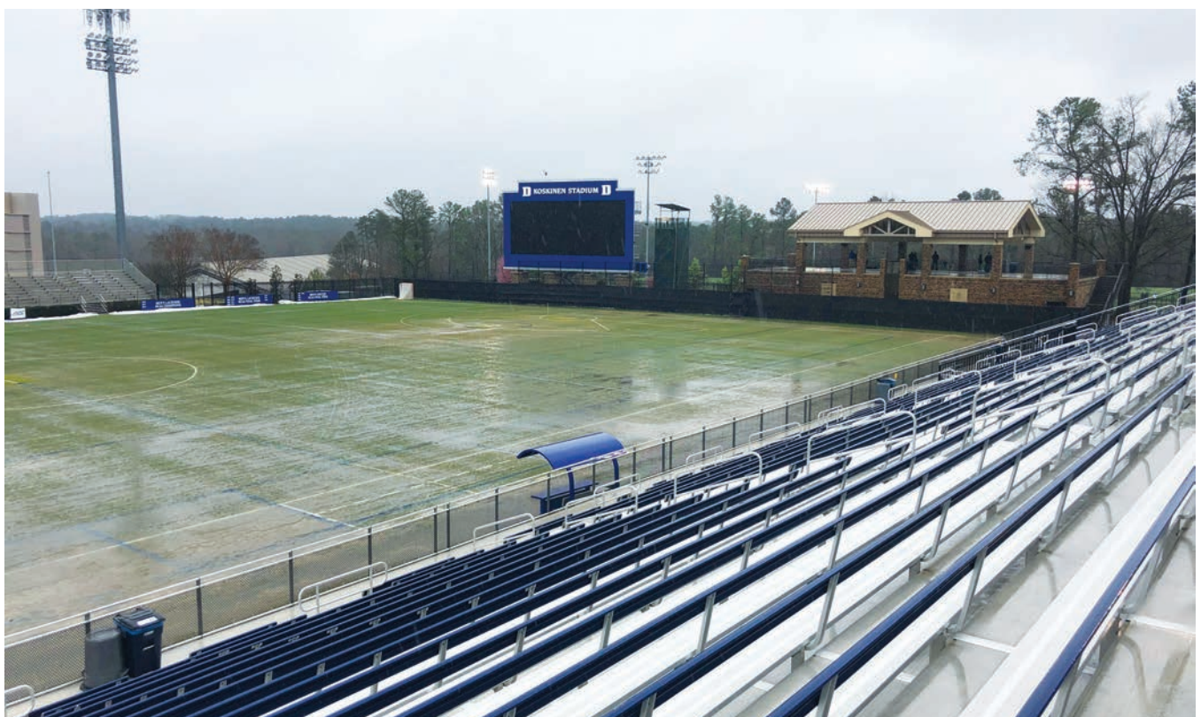
Pre-construction, drainage failure was on full display during the spring lacrosse season.
