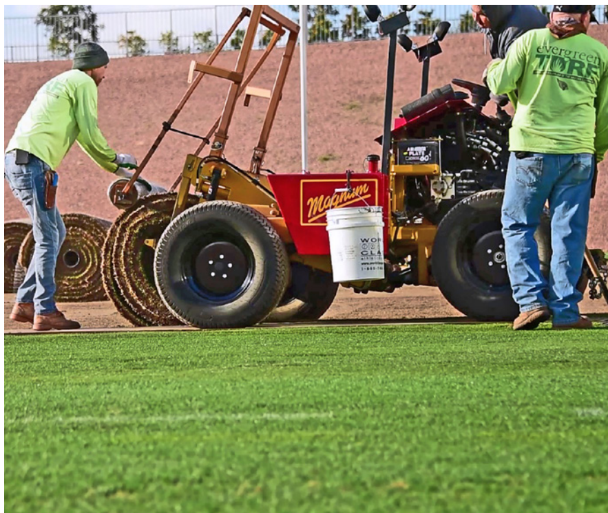
The Evergreen Turf crew is installing the thick-cut sod on the Arizona Cardinals moveable field outside of State Farm Stadium. Photo courtesy of Jimmy Fox, Evergreen Turf
