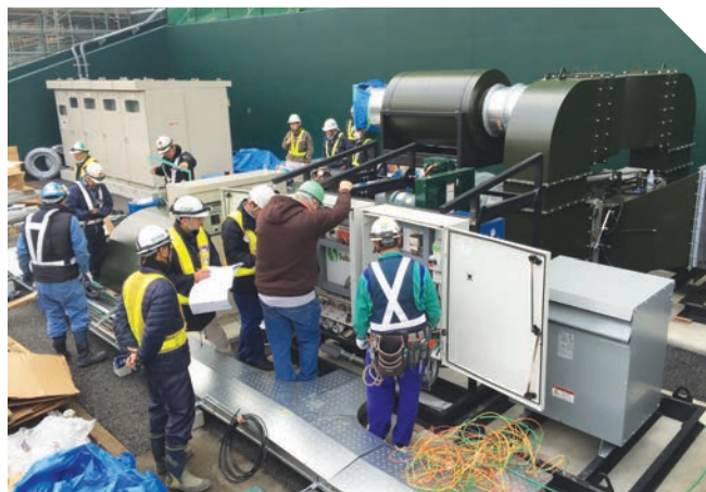
A SubAir Sport system being installed in Japan.
