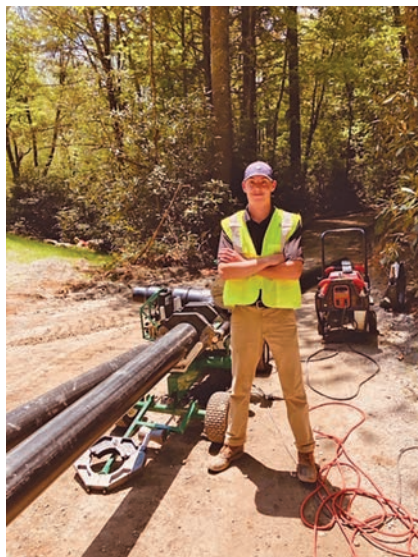
Horry-Georgetown graduate Chandler Hartwell setting up fusion for large mainline. Once fused, the pipe will be dragged to the installation area. No damaged to the pipe occurs from dragging and it can't pull apart. Both would be issues with PVC.
