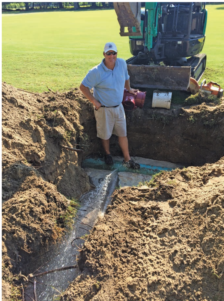
The author standing over a leaky PVC pipe that he's waiting to drain down so that he can repair it.
