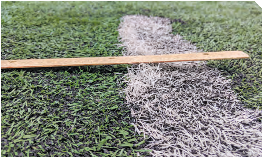
Separating or uneven seams and inlays should be fixed using manufacturers' recs.
