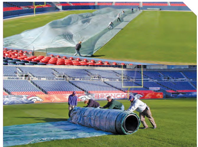
Covers can be folded in successive halves and rolled up onto a drum for removal and storage. ©Ross Kurcab, CSFM
