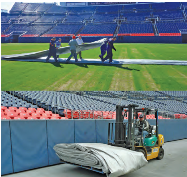
Large area covers can also be folded lengthwise and placed on a smooth-topped pallet for careful removal with forklift. ©Ross Kurcab, CSFM.
